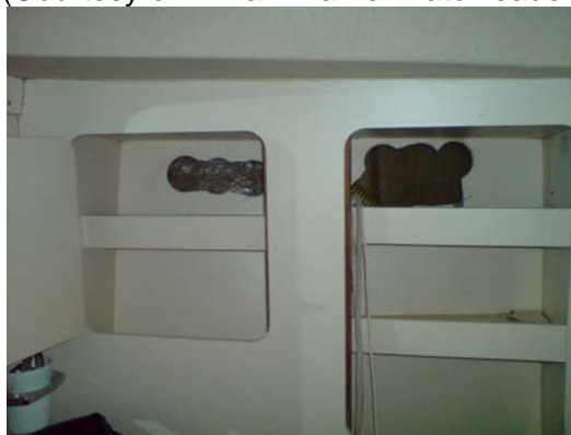
Holes cut in Upper heads lockers. (CUT THE AFT ONE FIRST)
